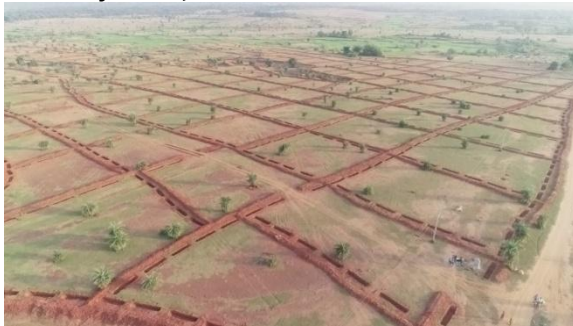
Construction of Trench cum Bund (TCB)
