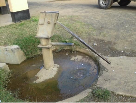
Auto flow well at Primary School, Pokharia West, Sikaripara block, Dumka
