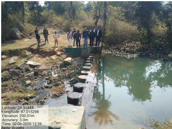
Construction of check dam
