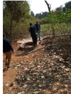
Construction of soak pit
