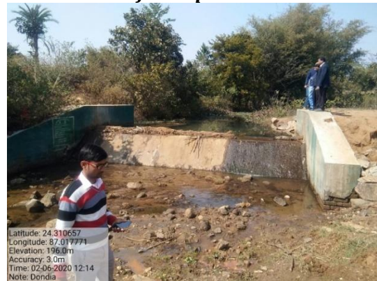
Construction of check dam
